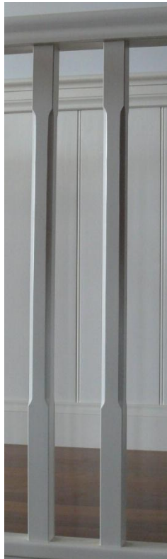
Stop chamfered balusters (for paint finish)
